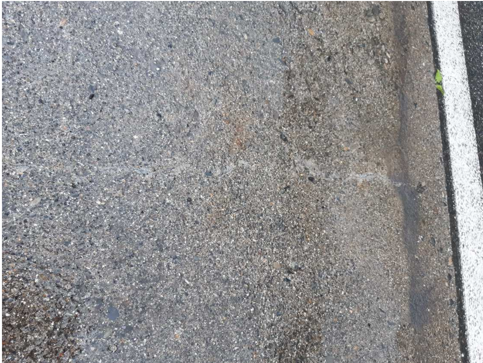
Figure 57 : fissure transversale – RD aval
