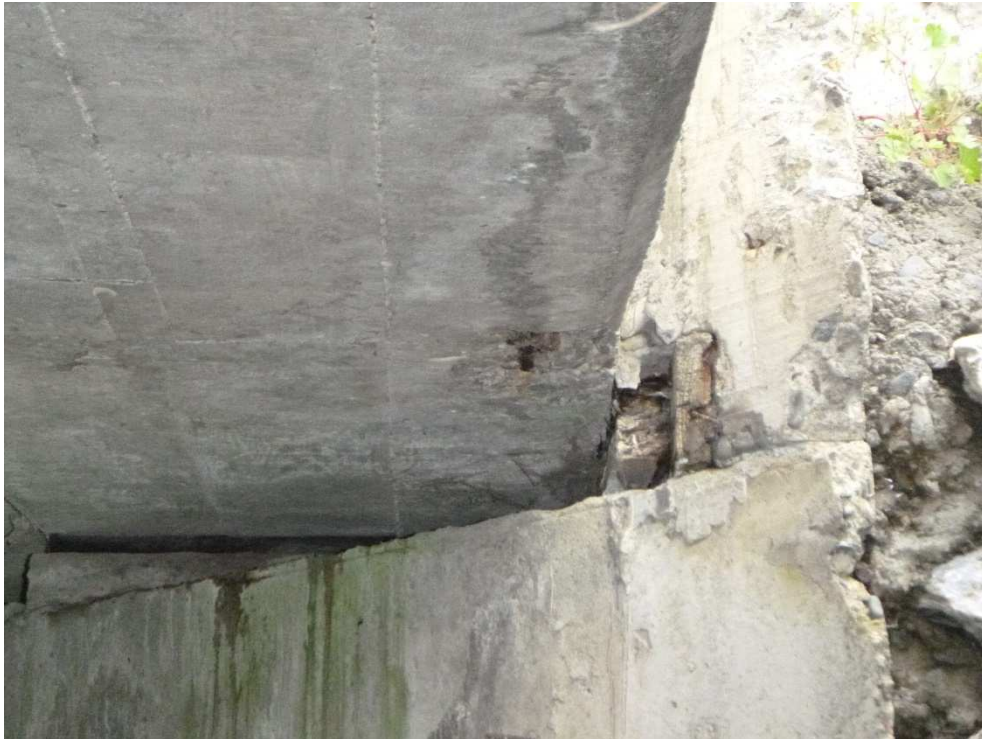
Figure 25 : pt1 – acier apparent corrodé – RD amont
