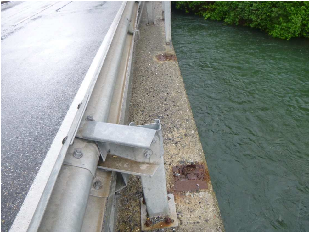
Figure 63 : absence de garde-corps – RG amont
