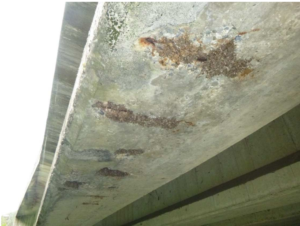
Figure 26 : pt1 – acier apparent corrodé – milieu de portée, aval
